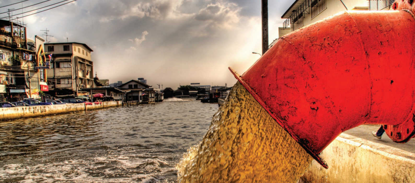
Égouts. Photo/Trey Ratcliff Creative Commons
