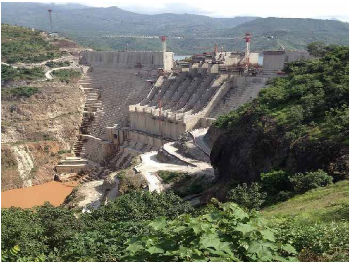
Figure 27. Gilgel Gibe III – a controversial hydroelectric dam in Ethiopia
